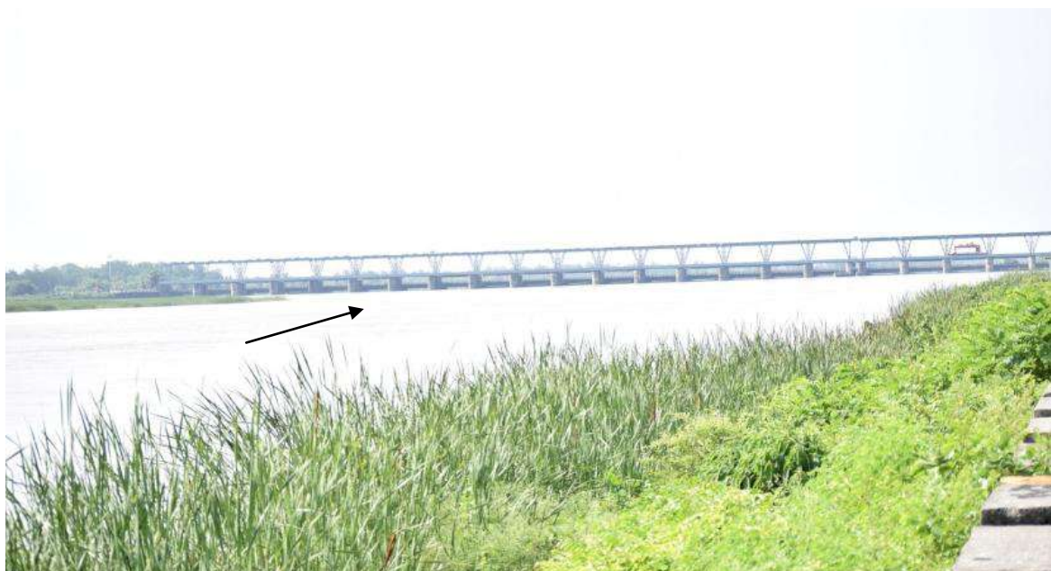
Figure 4.2 Sharda river at Banbasa barrage
