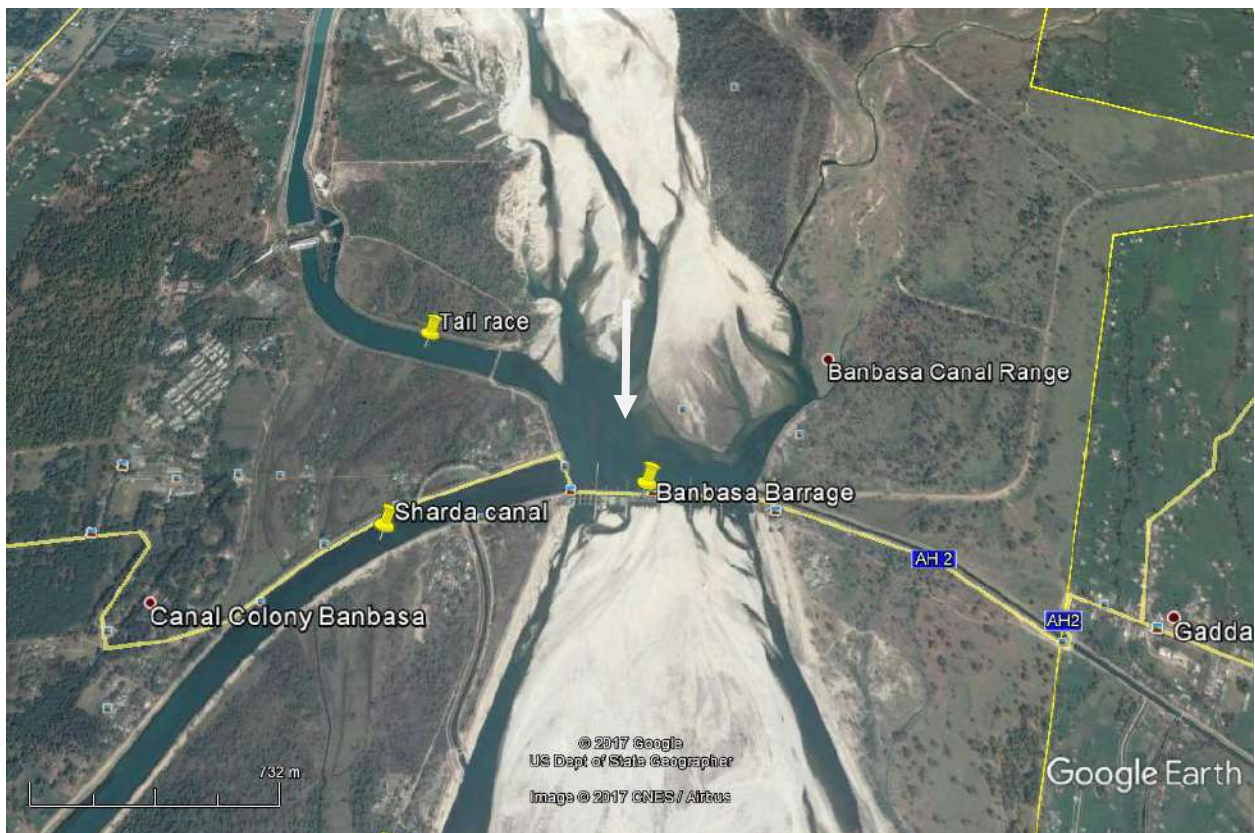
Figure 9.3a Location of the Banbasa barrage
