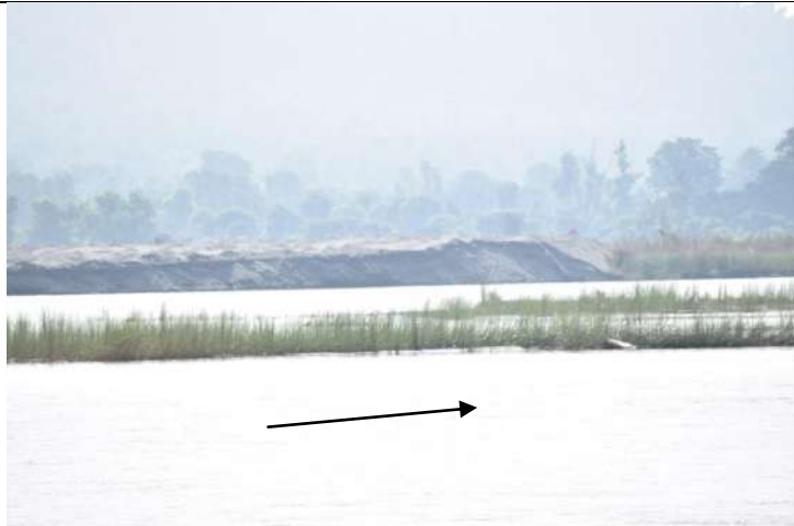
Figure 10.4 Right bank erosion upstream of the Tanakpur Barrage
