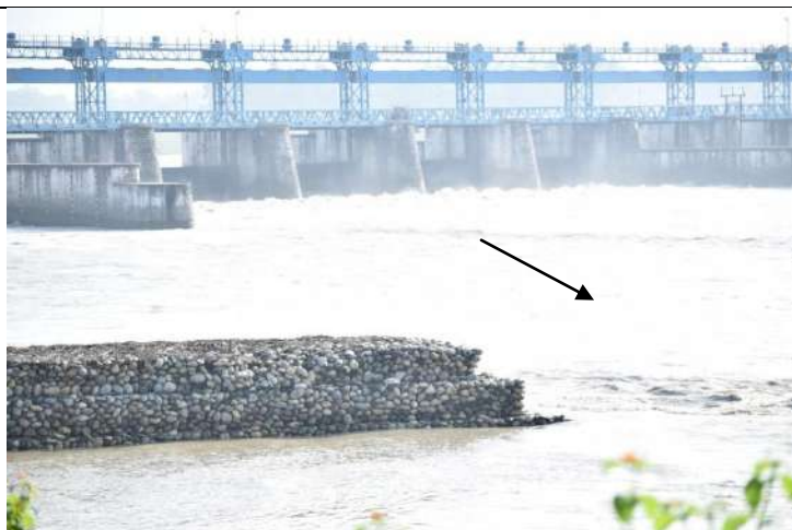
Figure 10.2 A spur on right banks downstream of the Banbasa barrage
