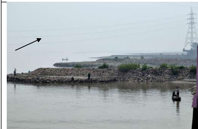
Figure 10.12 Series of spurs along right bank downstream of the Sharda Barrage
