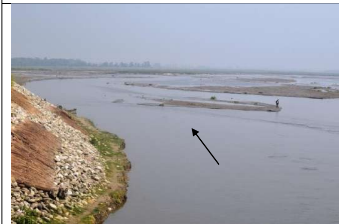
Figure 10.15 Downstream view of the river from road bridge at Palia Kalan
