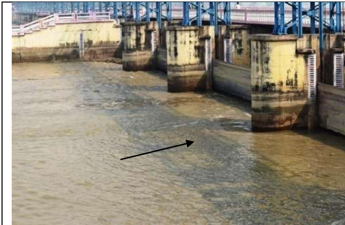
Figure 10.10 Upstream view of the Sharda Barrage
