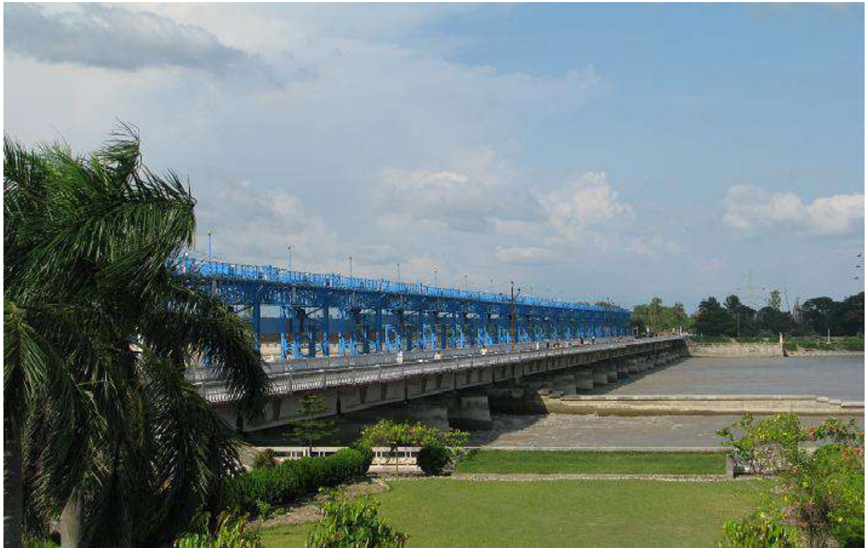
Figure 9.5b A photograph of the Lower Sharda Barrage
