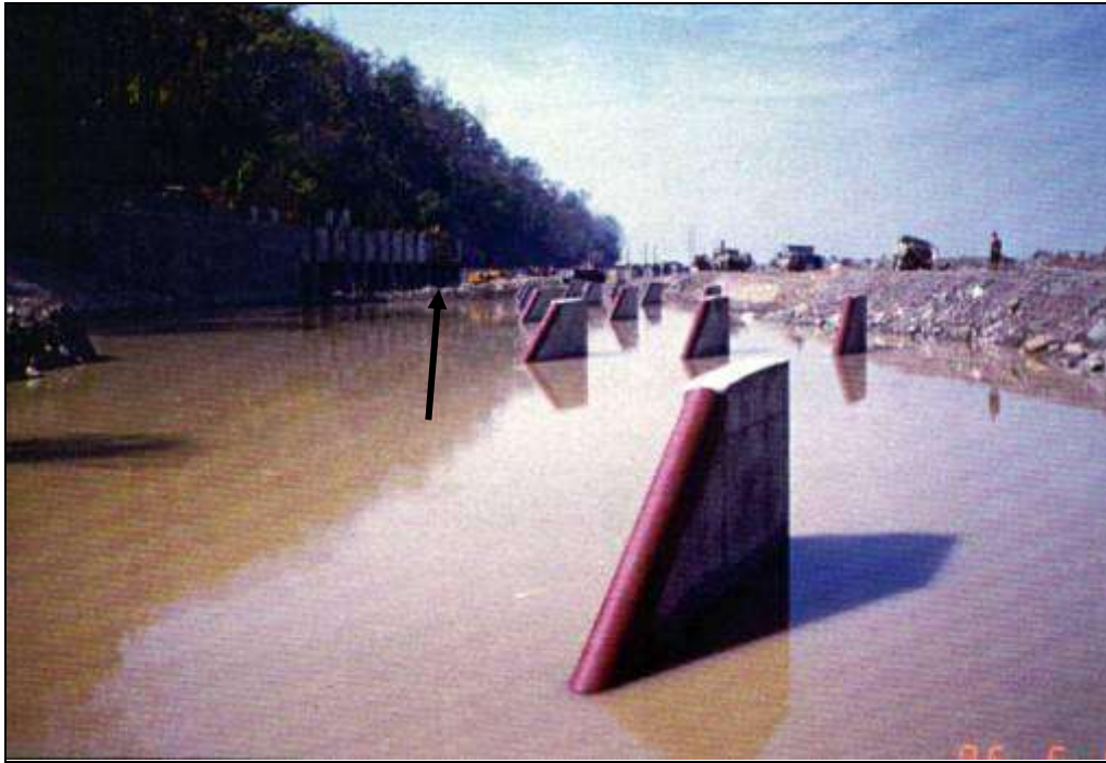
Figure. A13 Vanes installed at a water intake on Kosi river, Nepal
