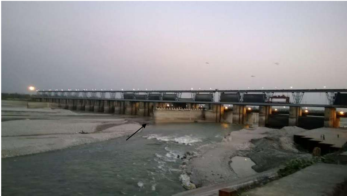
Figure 9.1b A photograph of the Tanakpur Barrage
