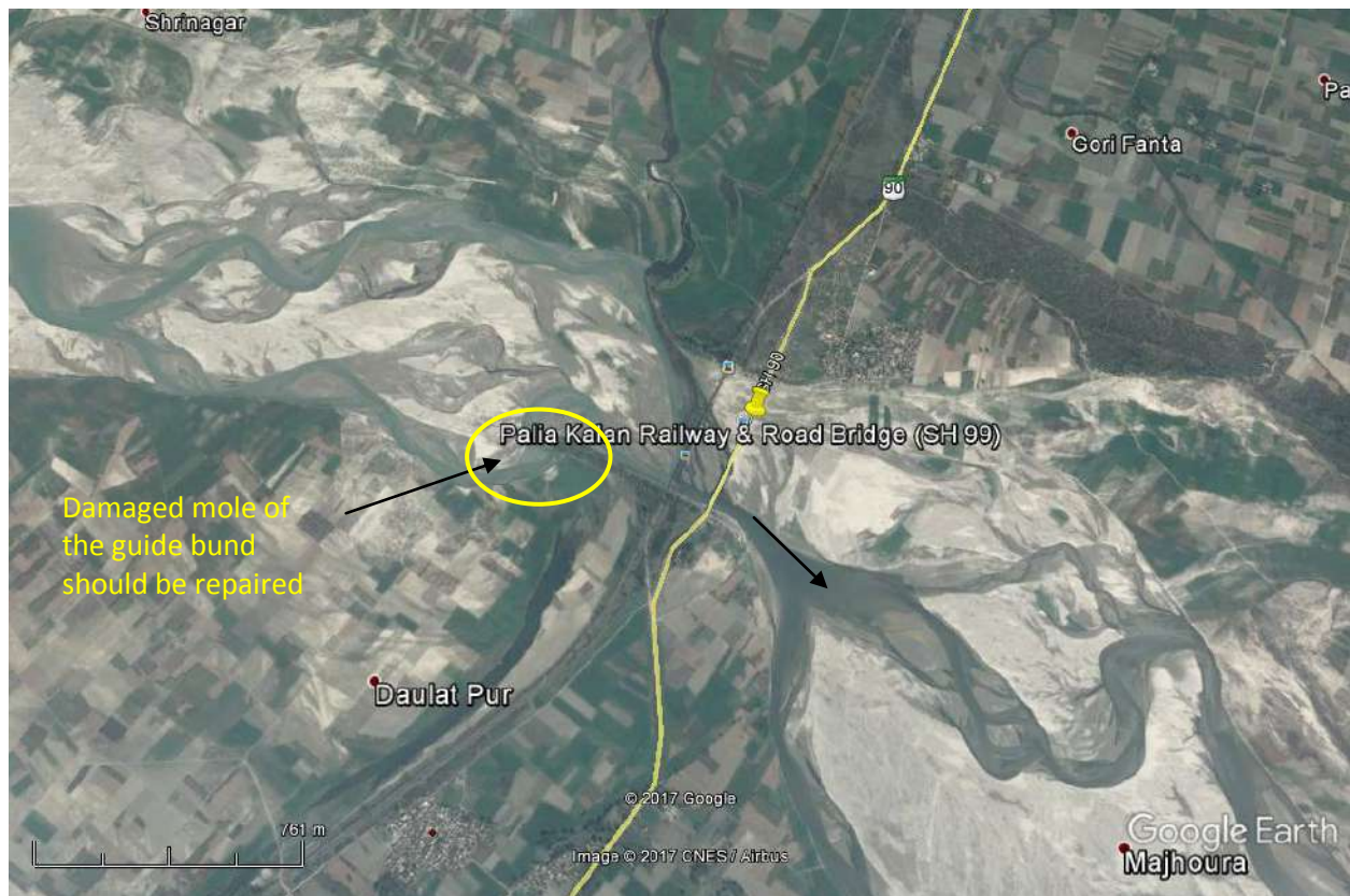
Figure 9.7 Location of Road (SH 90) cum Railway Bridge at Palia Kalan
