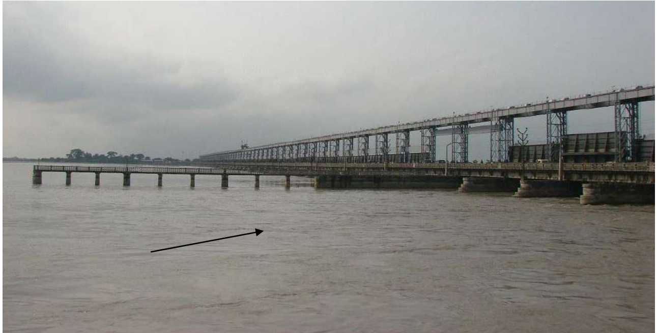
Figure 9.3b A photograph of the Banbasa Barrage (chainage 269 km)
