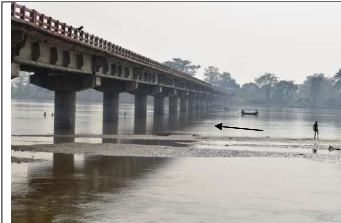
Figure 10.14 Road bridge on State Highway No. 90 at Palia Kalan
